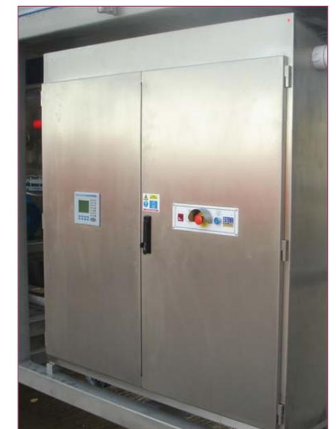
Stainless steel control panel with PLC control
